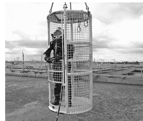
crawling through a tub of rotting cottage cheese, at 40 degrees". Major works have also been conducted at the same plant to relocate piping inside the reactor and to dredge and remove approximately 1000 cubic metres of dead bacteria, from the floor of the reactor.
